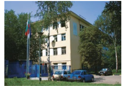
Elprom ZEM production plant
