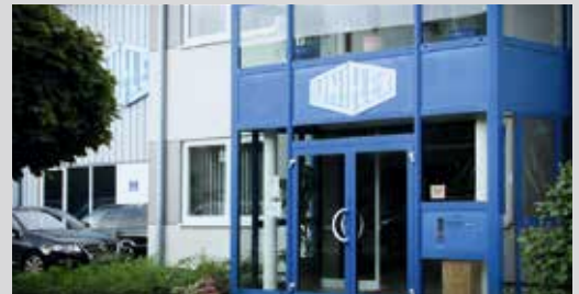
UNIFLEX moves into a bigger office and production facility in Karben, 10 km north of Frankfurt
