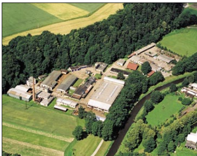
Production plant of the company Kostelec nad Orlicí
