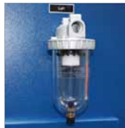
WATER SEPARATOR for pressure air
